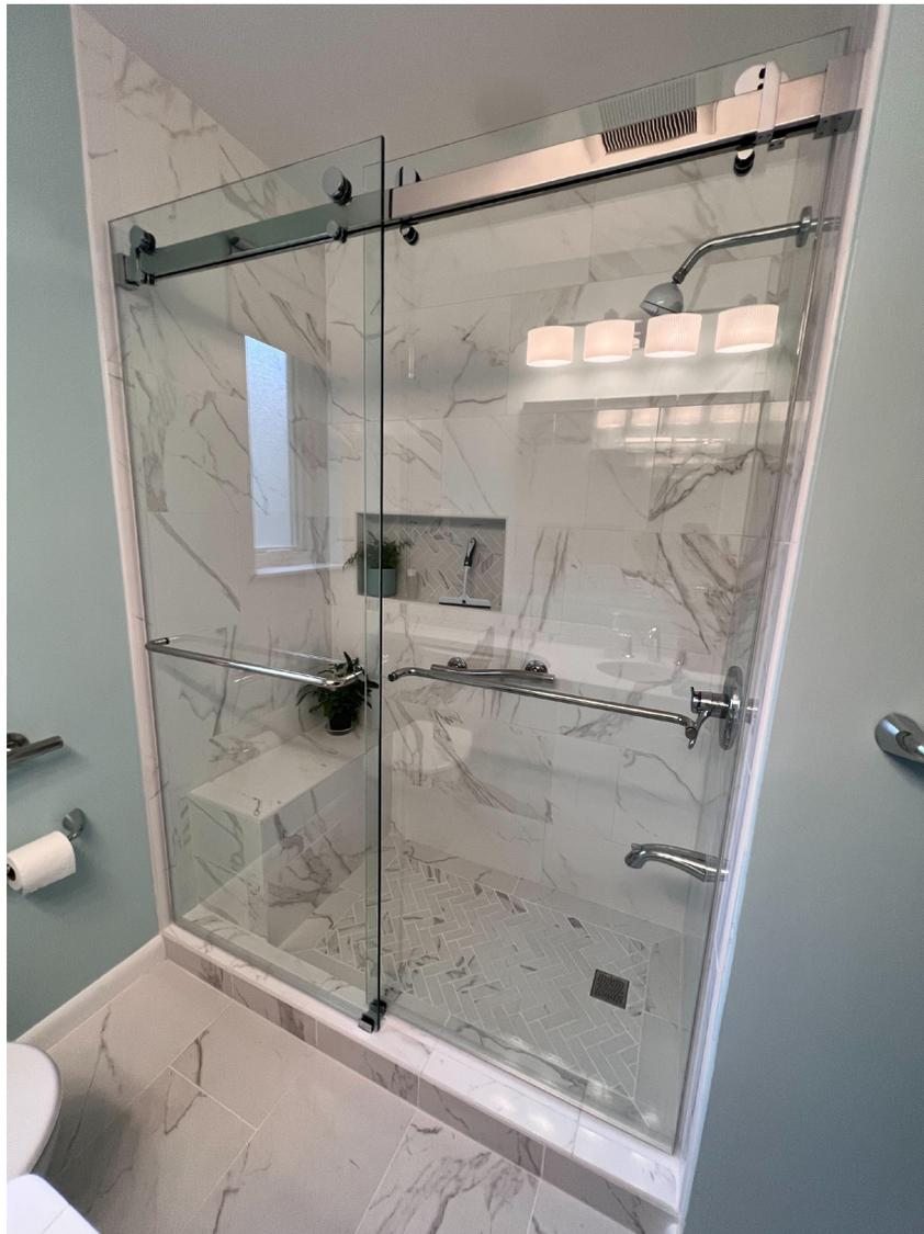
\*\*\*Notice there is no vertical metal on the sides or horizontal metal on the bottom, as you would find in box stores. While this eliminates adjustability, it adds to the customized fit and finish, clients prefer.\*\*\*
